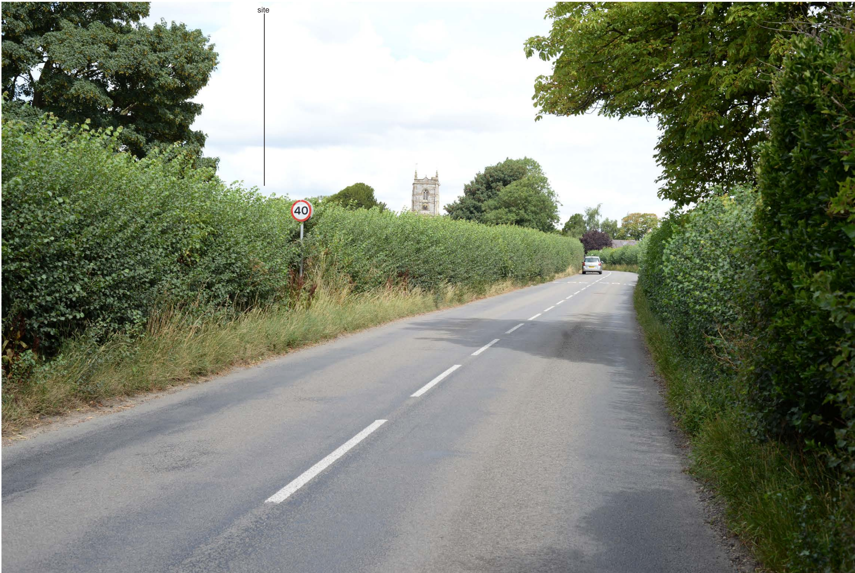
Viewpoint 10 Looking north on the B3092 towards St Gregory the Great church tower approximately 12m away from the site boundary
